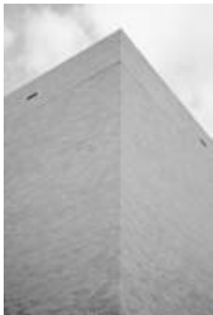
Figure 10-56 Differential expansion between parapet and building wall.
