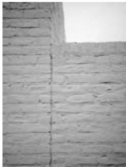
Figure 9-16 Expansion joint at change in brick wall height.
