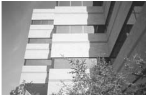
Figure 10-65 Strong horizontal color bands disguise wide soft joints at shelf angles.
