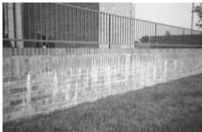
Figure 16-5 Calcium carbonate stain.
