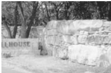
Figure 10-24 Dry-stack wall with large and small stones.
