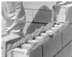
Figure 15-15 Fill head joints for better resistance to rain penetration. (From BIA Technical Note 17C.)
