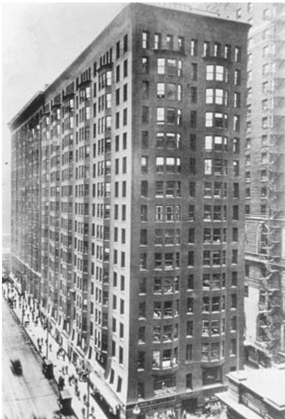
Figure 1-2 The Monadnock Building in Chicago (1891, Burnham and Root architects) was the last unreinforced high-rise masonry building. (Photo courtesy of the School of Architecture Slide Library, the University of Texas at Austin.)
