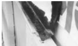
Figure 9-33 Lap moisture-resistant membrane over flashing.
