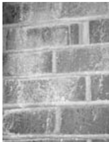
Figure 16-2 Efflorescence.
