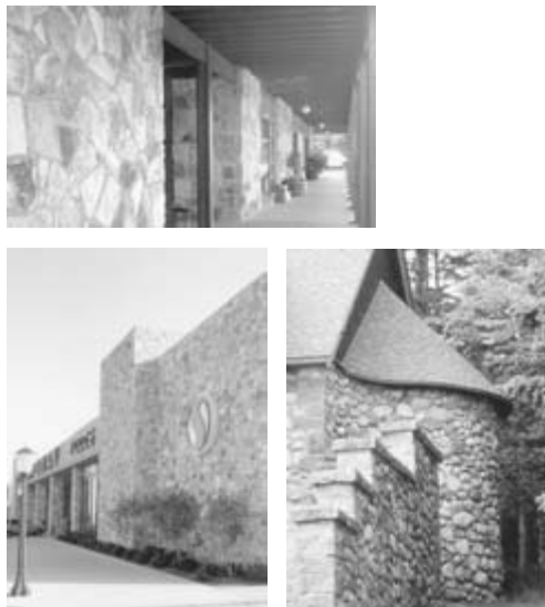
Figure 5-11 Rubble stone veneers.
