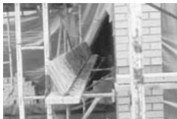
Figure 15-58 Turn scaffold boards on edge at the end of the day to avoid splashing mortar droppings or dirt onto the face of the wall.
