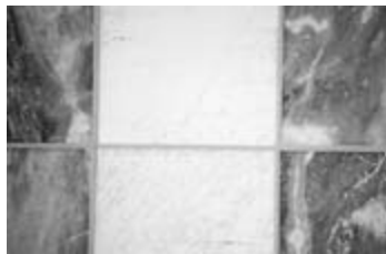
Figure 10-51 Elastomeric sealants are used instead of mortar at the joints of stone cladding systems.
