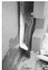
Figure 9-33 Lap moisture-resistant membrane over flashing.
