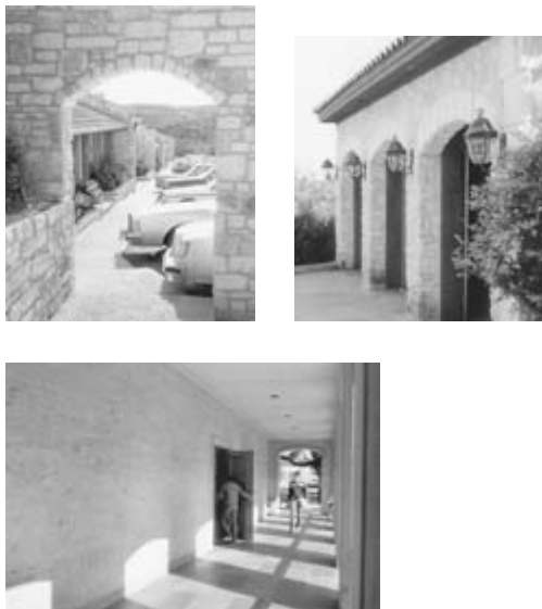
Figure 10-48 Mortar-bedded stone veneer.
