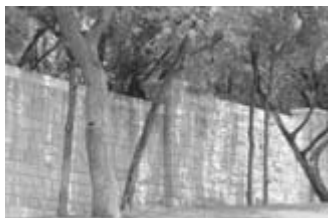
Figure 10-24 Dry-stack wall with large and small stones.
