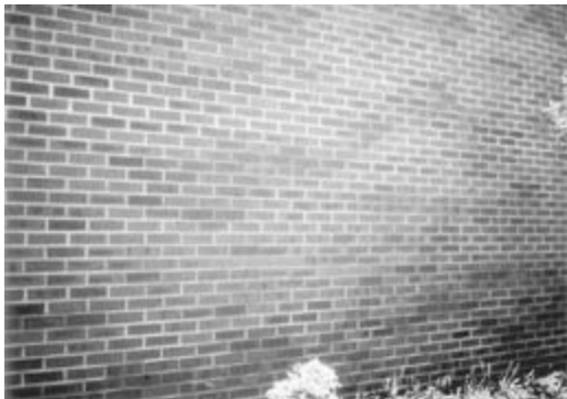
Figure 15-25 Joints should be tooled at a consistent moisture content because drier mortar tools to a darker color than mortar that is wetter when tooled.
