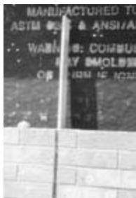
Figure 15-40 Brick masonry expansion joints.
