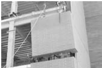
Figure 15-59 Lifting a prefabricated masonry panel into place.
